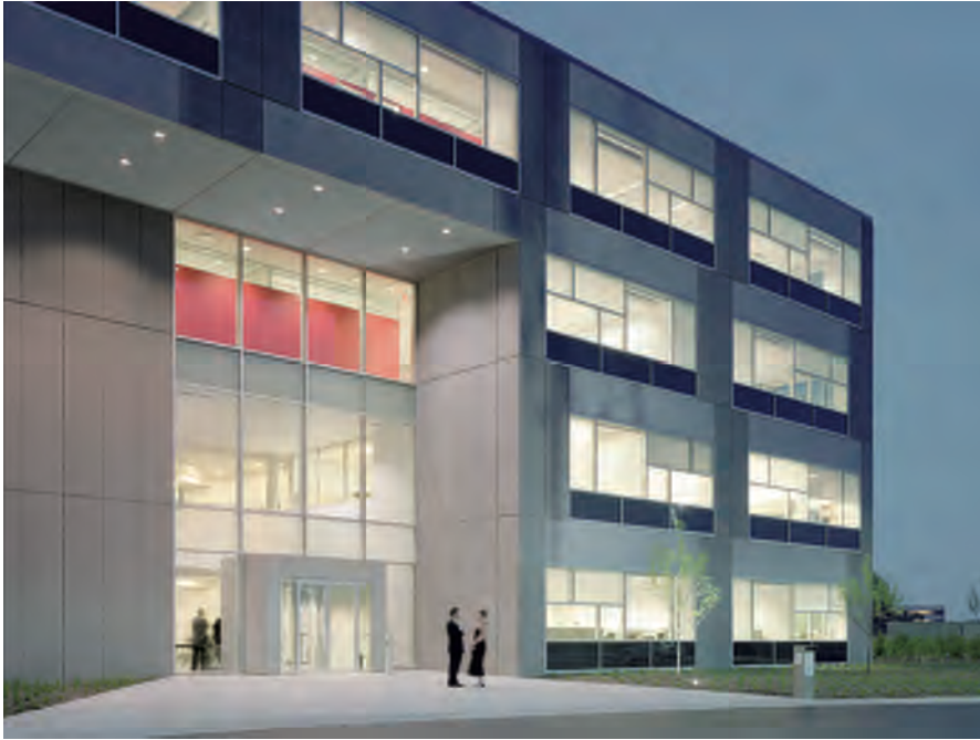
Irwin Mortgage Headquarters in Indianapolis, Indiana
